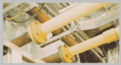
Claymore accommodation area, a 3" bore pipe was used where normally a 4" Cunifer pipe would be required. This was an added benefit because the complex arrangement of pipes and service ducts. With the handling so easy, long sections could be assembled in corridors and lifted into place without much effort or the use of special equipment.
